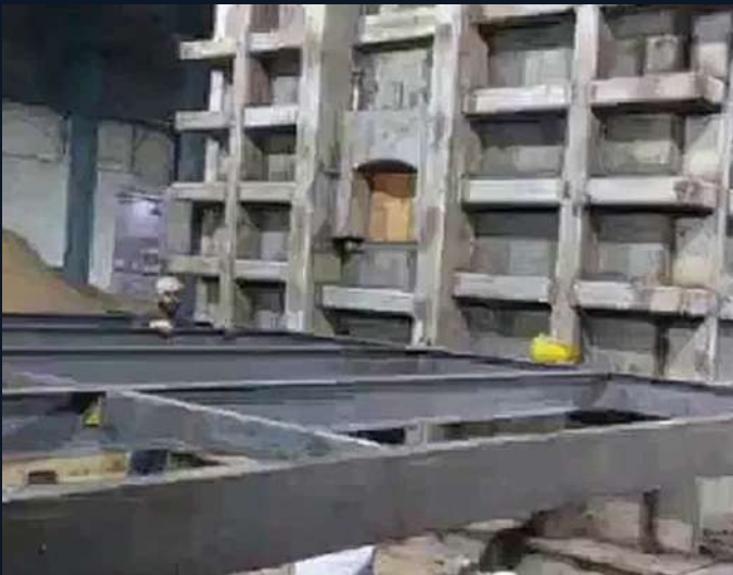
Furnace Fabrication and Installation
