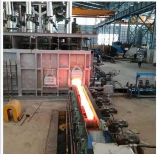
Billet Reheating Furnace | Handling section
